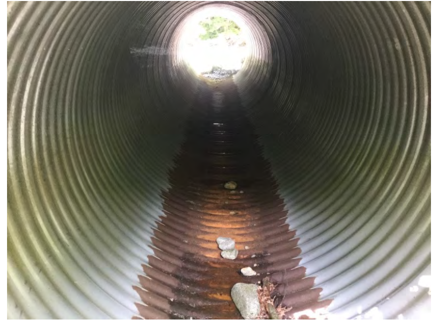
Clean through the low chain culvert
